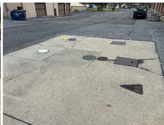
Underground storage tanks & drainage area
