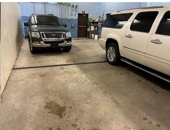
Township Vehicle Wash Bay
